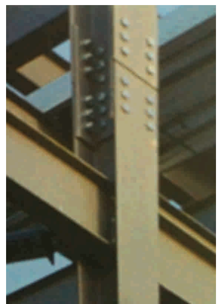
Splices inside makes structures aesthetically more appealing
